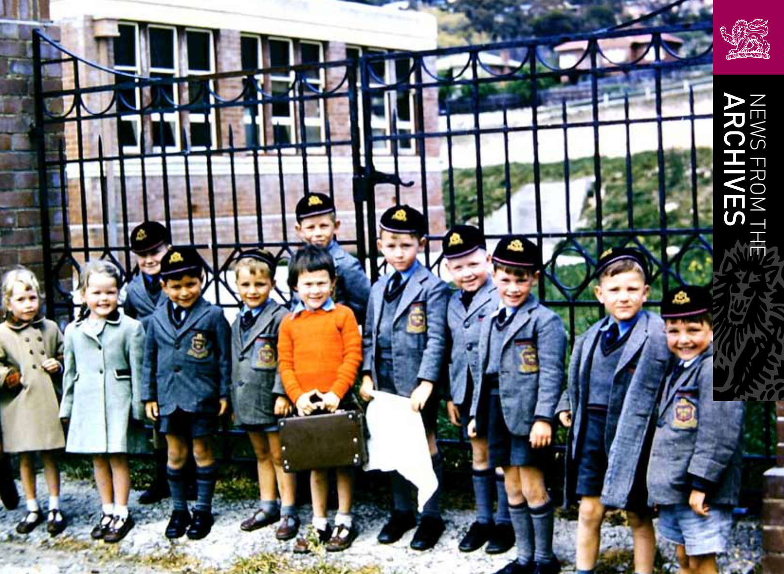
David Avenue entrance, 1957.
